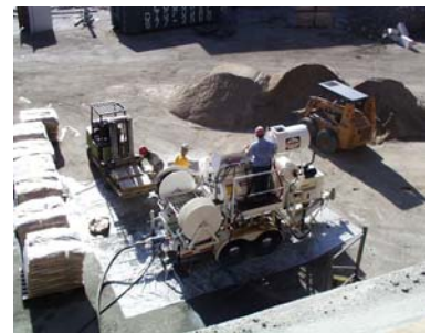
Pumping the floor product
