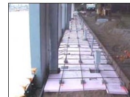
Prepping for the dock slabs.
