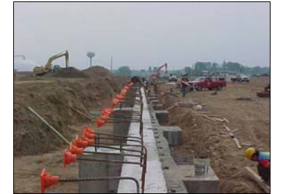
Pouring foundation walls.
