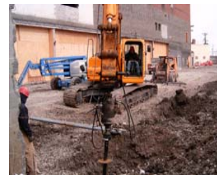
Excavator installing a helical pier starter adjacent to an existing building.
