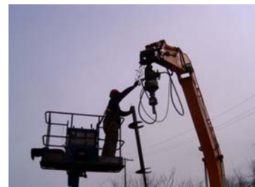
Keith Morse in a manbasket hooking up a 21' extension.
