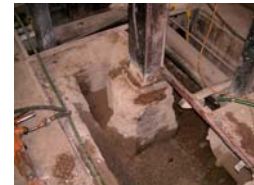
Concrete pedestal and steel column as surrounding concrete floor is removed.
