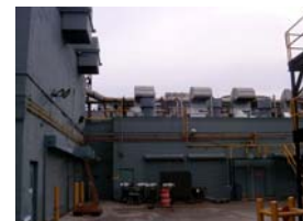
Test Cell area with second story penthouse in the background.
