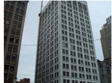
The Kales Building
