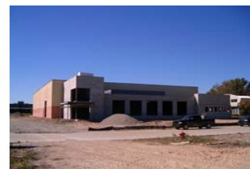
One of the buildings under construction.
