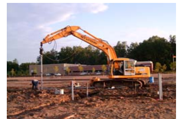
Installing a starter section.
