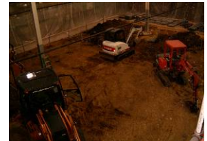
Installing piers and excavating around columns.
