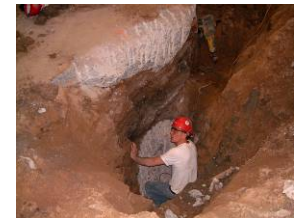
Footing preparation to install plate pier brackets.
