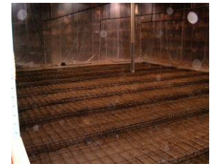
Reinforcing for structural slab.
