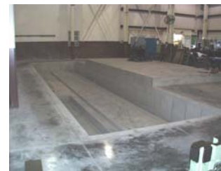
The finished product - a custom built high tolerance mill foundation
