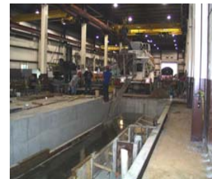
This machine base is 43’ long and super flat
