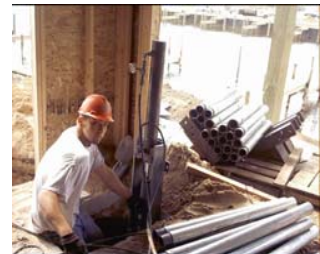
Cliff installing resistance piers on foundation
