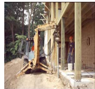
Backhoe installation of helical piers
