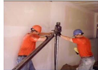
Tim and Rex installing floor helicals
