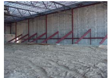
Ice arena seating risers on concrete foundations.
