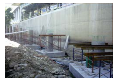
Support columns for river walk
