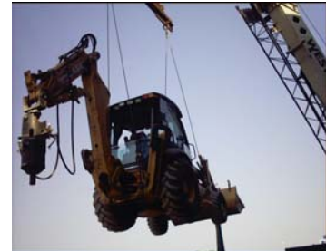
Crane lifting backhoe to the river bottom
